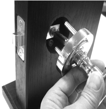
→5) Insert the remaining lock-half into the public (outside) side of the door. Note that the two threaded mounts on this lock-half insert into the larger tubes on the other lock-half.
