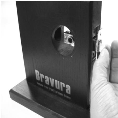
→ 2a) Insert latch mechanism into door. If using a privacy latch, make certain the threaded button is facing the side of the door from which you wish to lock the door (inside/non-public). Drill pilot holes for the latchbolt mechanism screws.
